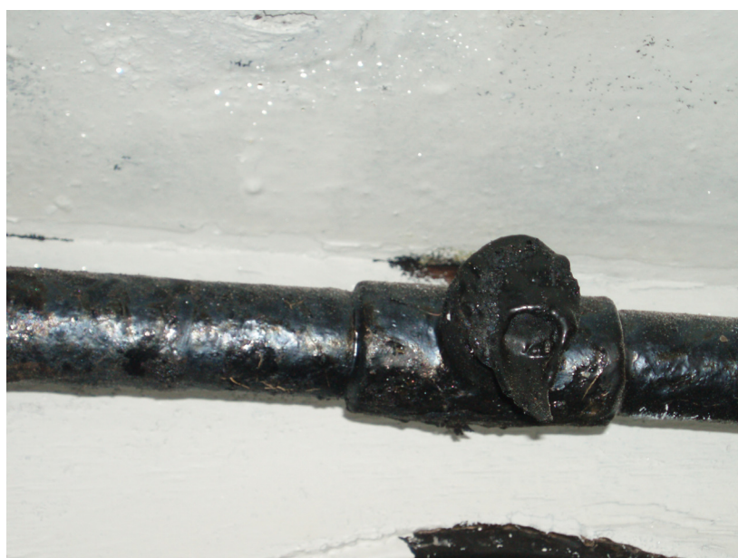
Plastic CO 2 discharge nozzle
