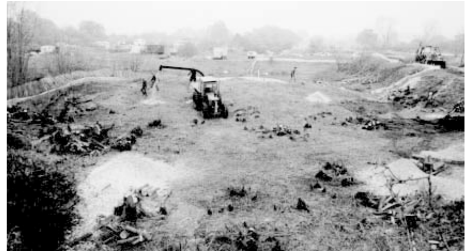
Plate 5 Shredding cut wood for mulch onsite re-uses natural local materials
