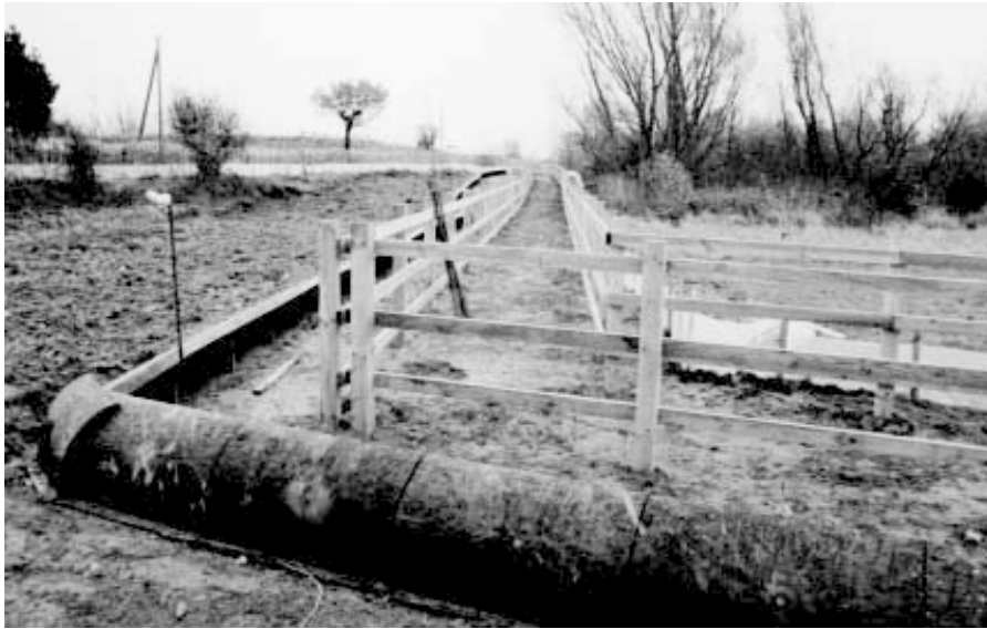
Plate 3 Fences to control amphibian movement and public access are often placed prior to final topsoiling, seeding and planting
