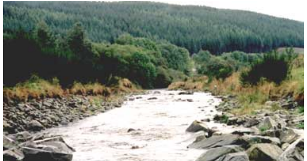
Evan Water River Diversion 2 years after construction: M6 Scotland
