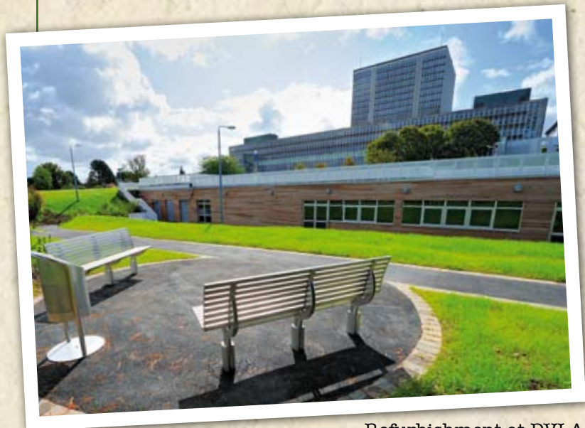
Refurbishment at DVLA
